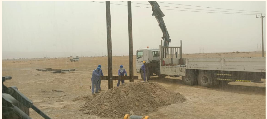
Unit Rate Tender No: 14/2022 in Al Dhahirah Governorate (ongoing)
